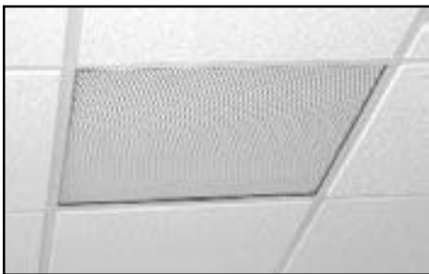
Figure 10: Completed subwoofer installation.
